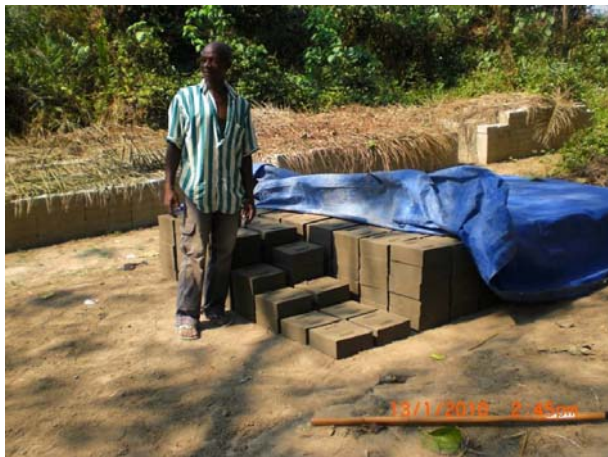
Over 15,000 blocks have been made for the school. The blocks set up best if kept somewhat moist and shaded, first by a tarp, and then by palm fronds.
