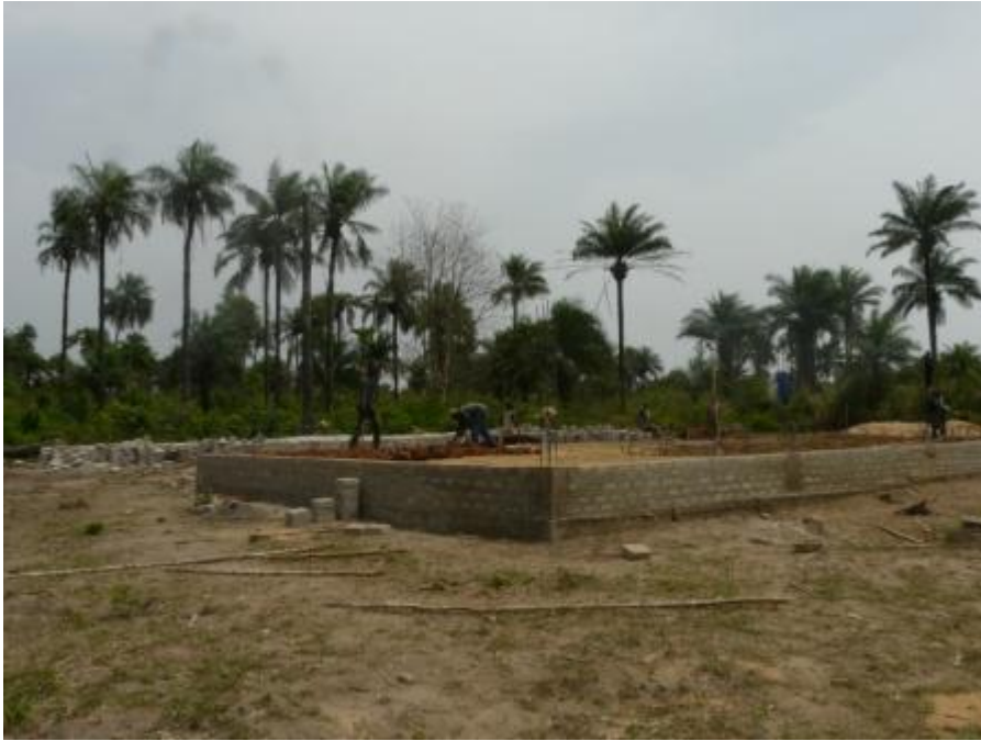
Beginning of the walls made out of the pressed and dried soil cement blocks.
