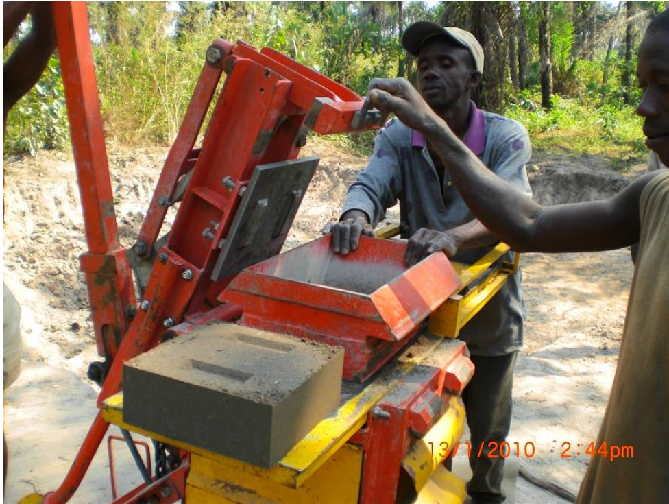
The press makes inexpensive blocks that are sturdier and more water resistant than the hand-made soil blocks usually used in Sierra Leone.
