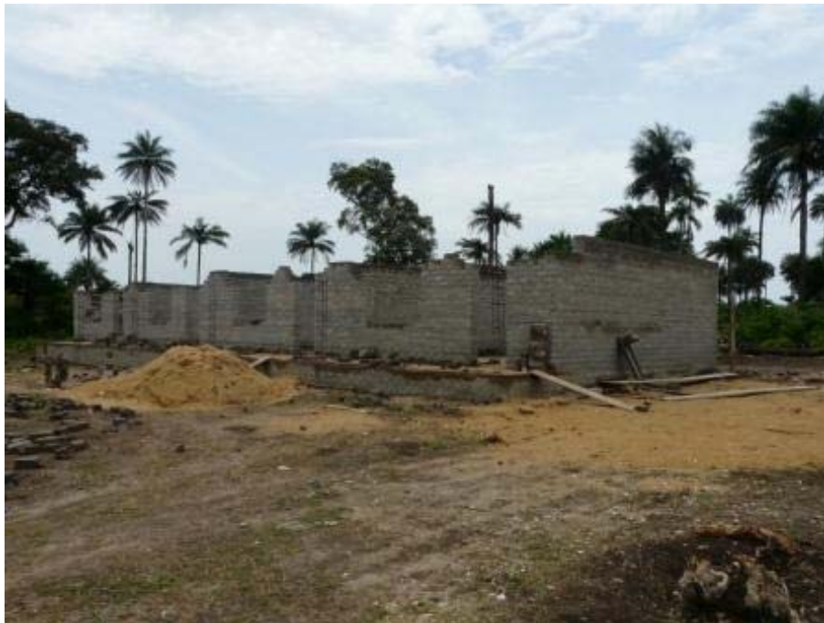
Beginning of the walls made out of the pressed and dried soil cement blocks.
