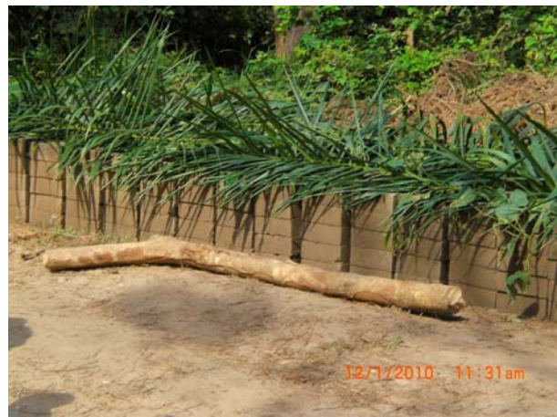
Over 15,000 blocks have been made for the school. The blocks set up best if kept somewhat moist and shaded, first by a tarp, and then by palm fronds.
